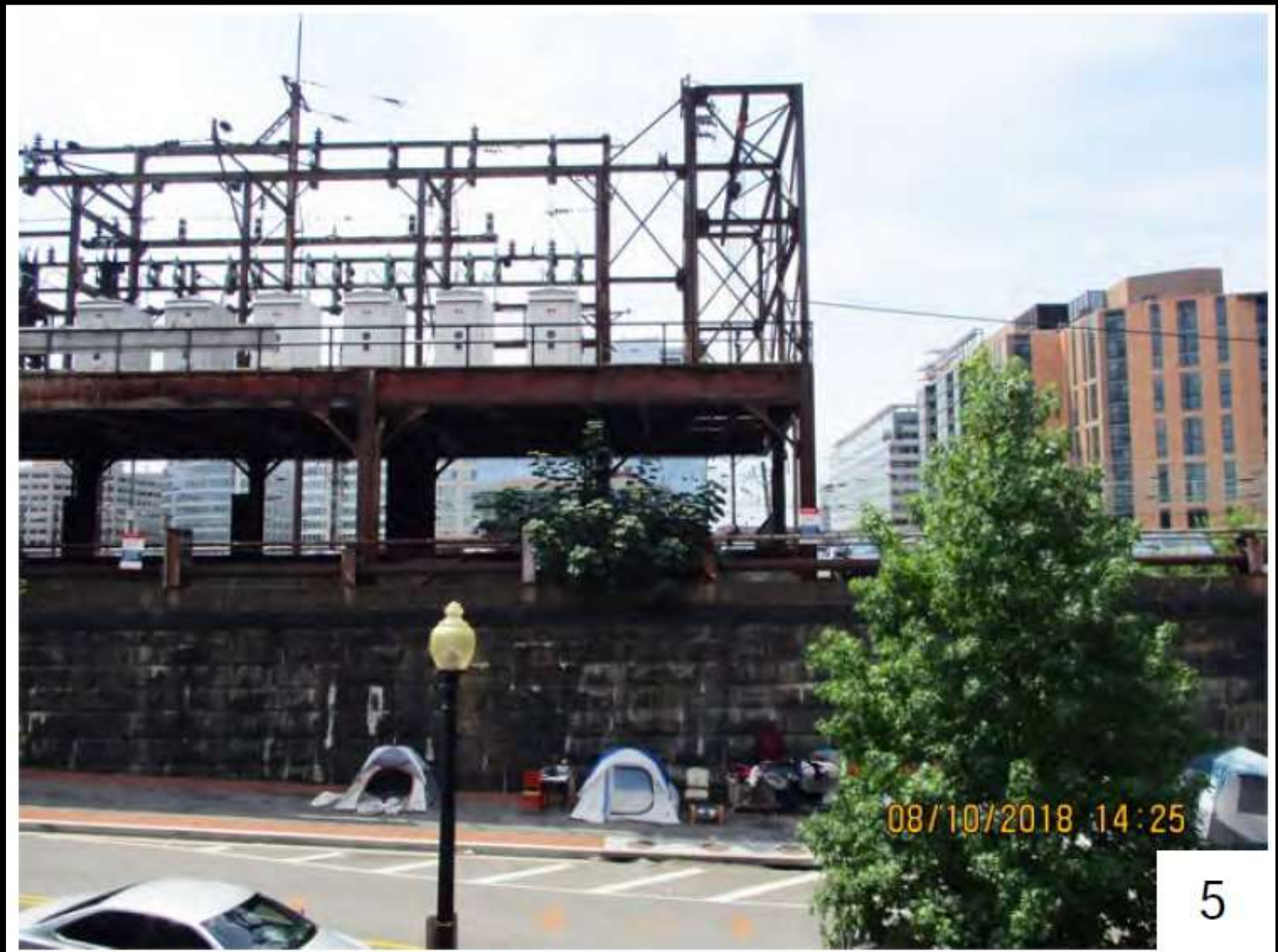
looking west from site at retaining wall & train tracks
